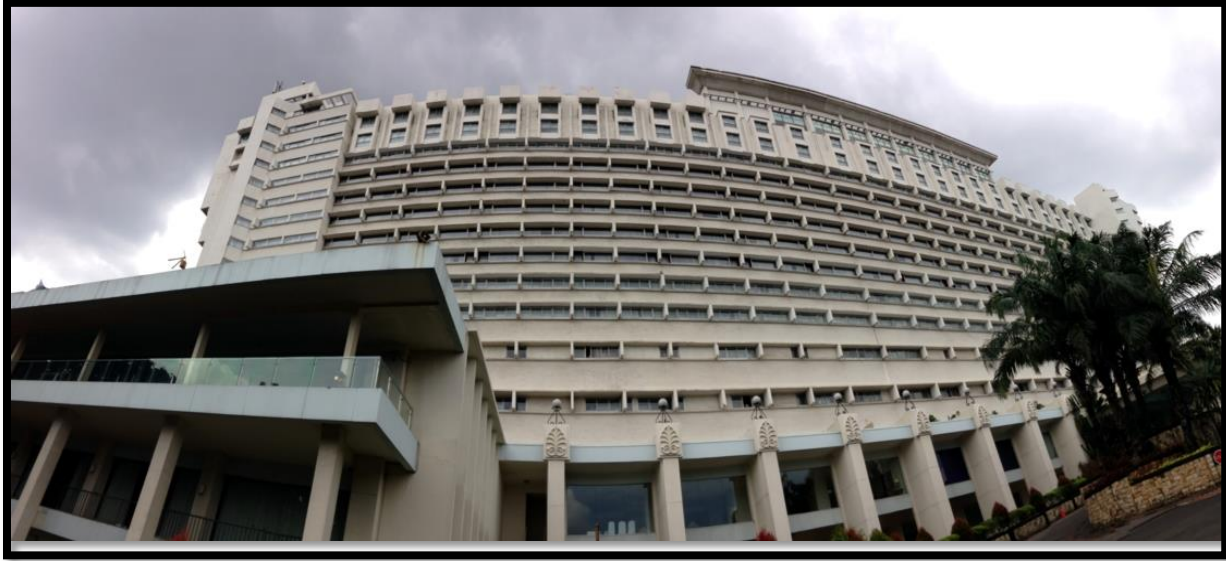
March 2015: A panoramic view of the front of the 5-star Hotel Borobudur in Jakarta, Java, Indonesia, which was formerly the site of "Bicycle Camp." (Photo: Dana Charles)
