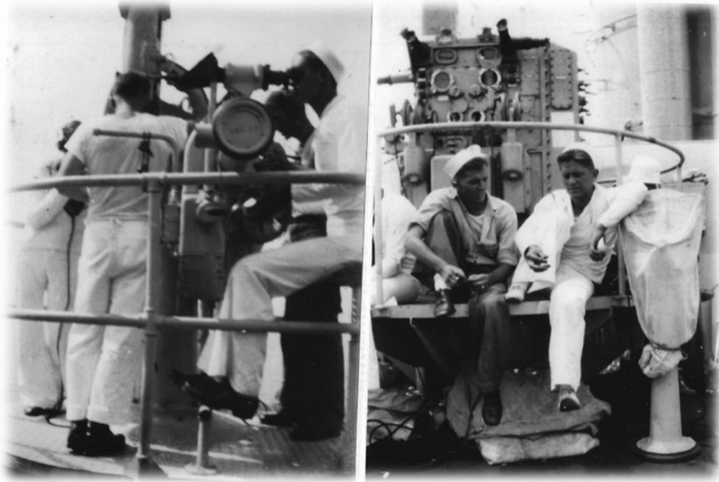
CA30's early MK19 Dual purpose directors were primitive & not very effective.
