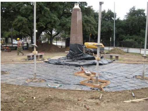
Beginning project: monument with old platform removed, base swathed for safety and layout for new platform and flagpole base.
